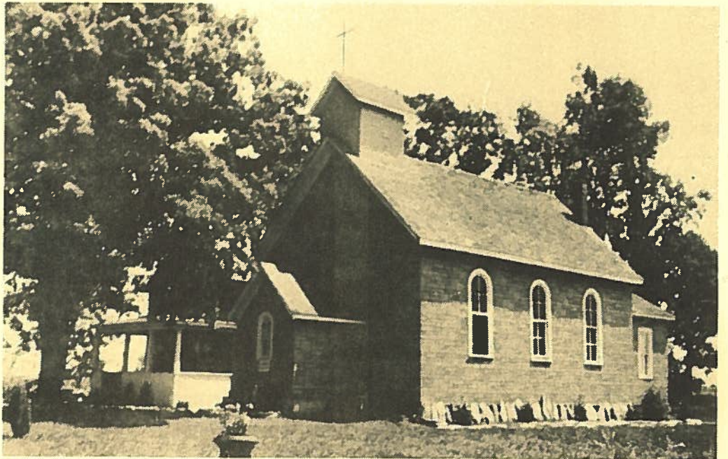
New insul-stone siding installed 1947
